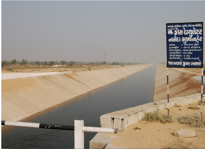
One of the many canals that make up the SSNNL canal system.
