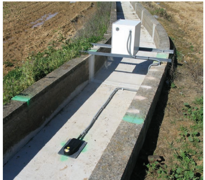
SonTek/YSI Argonaut-SW deployed in an irrigation canal.
