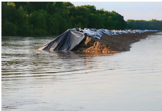
A dedicated vertical beam in the new SonTek RiverSurveyor allowed researchers to precisely map the bottom of a break in this Mississippi River levee – vital insight into the performance of levees during the devastating 2008 flood.
